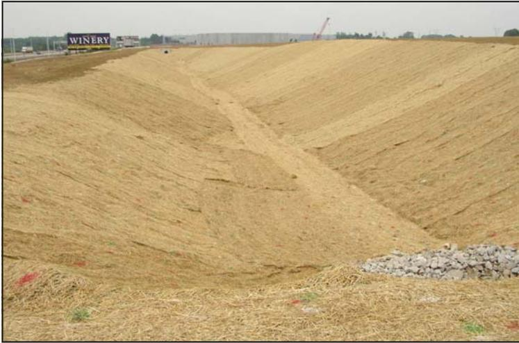
*An erosion control blanket is a biodegradable, organic or synthetic mulch incorporated with a biodegradable, photodegradable, or permanent polypropylene, natural fiber, or similar netting material. It is an alternative to mulch and normally used on slopes and in concentrated flow channels.*
