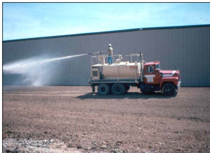
Figure 3: Hydroseeding
