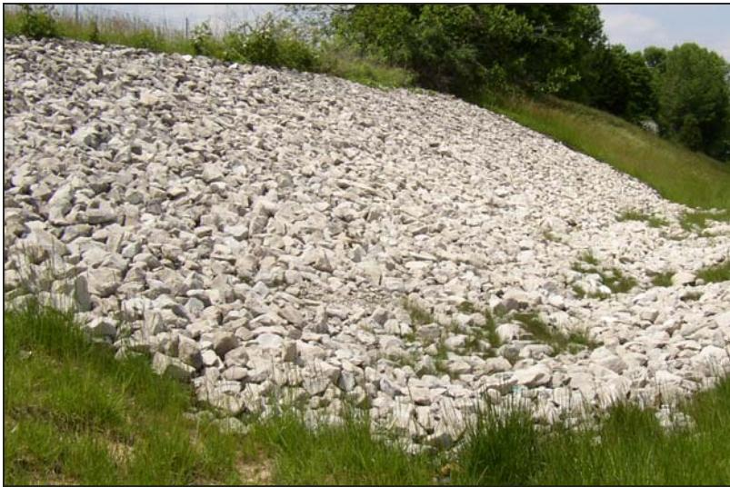
*Riprap slope protection* is an erosion control measure consisting of geotextile fabric and stone riprap that is placed on an unvegetated slope to protect the soil from erosive forces.
