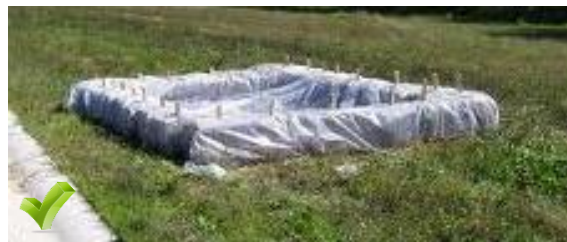
Good example of above grade system with straw bales and a polyethylene lining. A "Concrete Washout" sign should be installed at this location.
