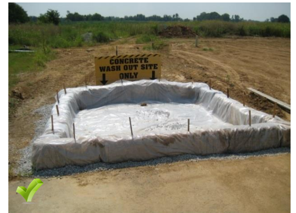
This above grade washout system has the correct polyethylene lining which is wrapped around the straw bales. The washout is underlain with DGA to provide a solid base for the washout and to prevent punctures in the plastic liner. Straw bales are securely anchored to the ground, and a large sign identifies the washout.
