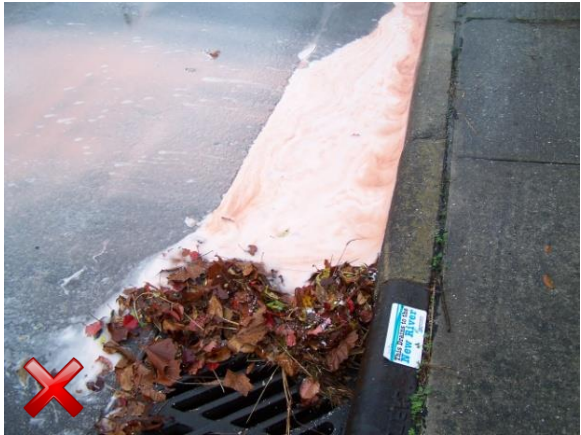
Suspicious color flowing into a storm drain is a good example of illicit discharge coming from some location nearby.
