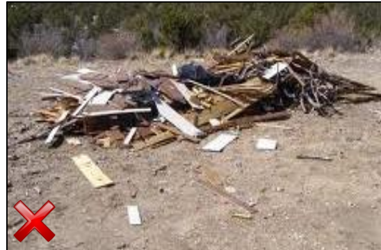
Properly dispose of construction waste into a provided dumpster. Pick up garbage to prevent items leaving the site. Make sure dumpster remains closed at all times to prevent exposure to rainwater.
