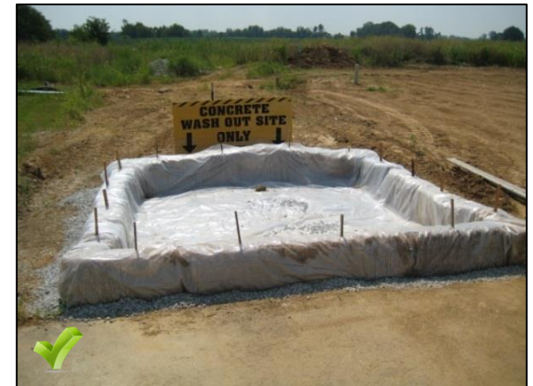
Contractors and subcontractors should utilize concrete washouts whenever pouring or placing concrete or mortar. Washouts should be used for rinsing off mortar and concrete mix on process and placement equipment. It is not acceptable to wash off equipment outside of a contained concrete washout area.
