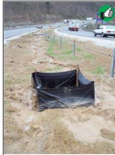
Good application of silt fence frame to protect inlet. Use wire fence backing to reinforce frame, or diagonal bracing across top of stakes. Make sure fence is trenched-in to prevent bypasses or undercutting. Inspect and remove sediment as necessary after each rain. Expect a more frequent replacement schedule for silt fence drop inlet protection.
