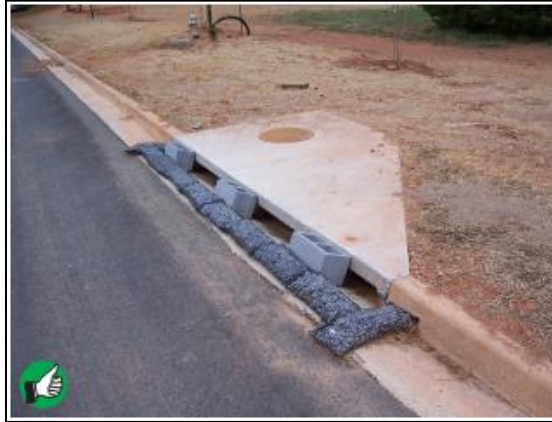
Excellent use of rock-filled mesh tubes to control sediment at curb inlet. Concrete block spacers keep tubes from moving into - and clogging - the inlet during heavy flows.
