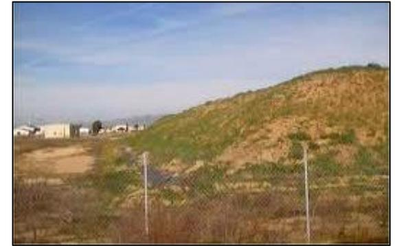
Stockpiles of soil can deliver large amounts of muddy runoff to paved roads, adjacent lawns, and local creeks. A silt fence should be placed around stockpile areas to prevent silt-laden runoff from leaving the site.
