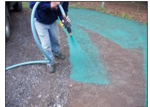
Hydro seeding applied to bare soil to speed up slope stabilization.
